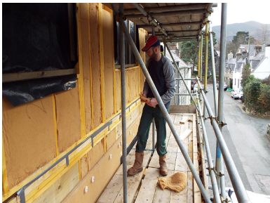
Company Director Gary Newman on site installing plant fibre
